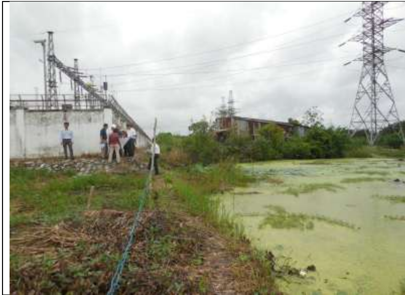
Fig 2a: Northeast corner of Binh Chanh substation from which new 220 kV transmission line will start. Existing 110 kV transmission line in background.
