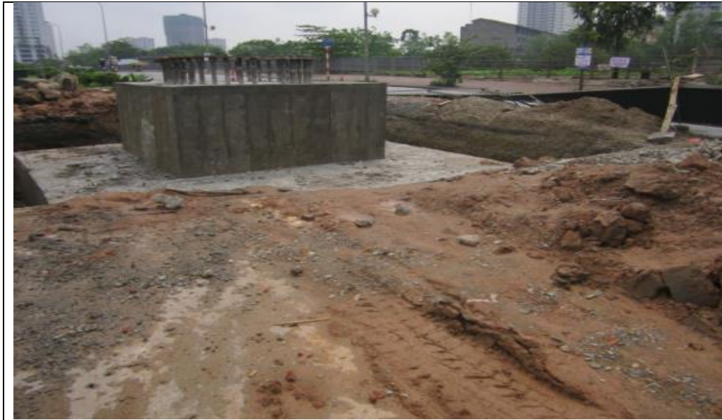
Pole No. 30 under construction
