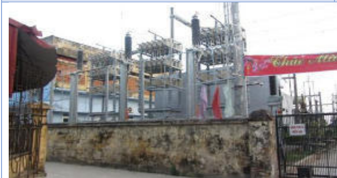
Photo 5: Position of Tía Substation
