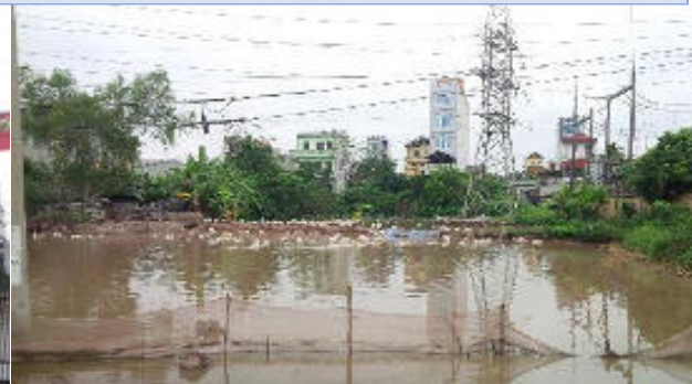
Photo 6: expanded area of Tía Substation
