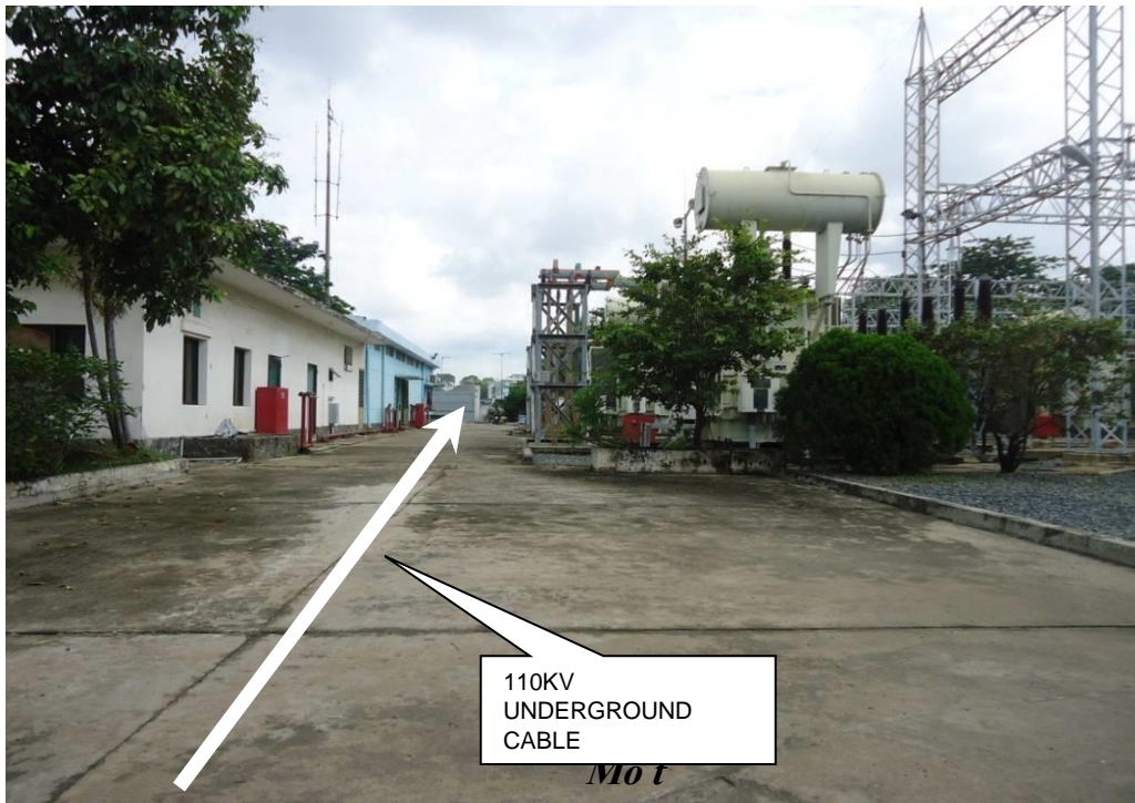
Picture 2: Description of the underground cables within the 110kV Chánh Hưng substation
