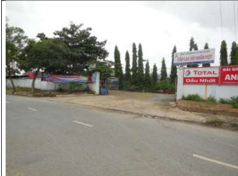
Fig 2e: Location of VINA Port Authority site where substation will be built
