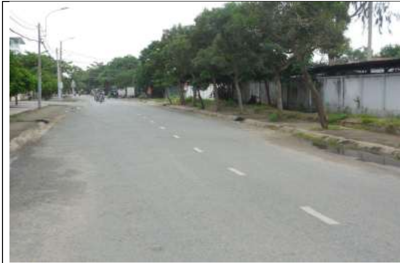
Fig 2d: Section of underground cable route beside new substation site
