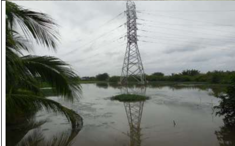
Fig 2b: Example 110 kV transmission tower that will be replaced with 220 kV tower, and underlying lowland flood area.
