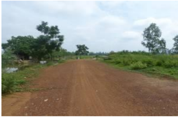
Access road – front view of the substation
