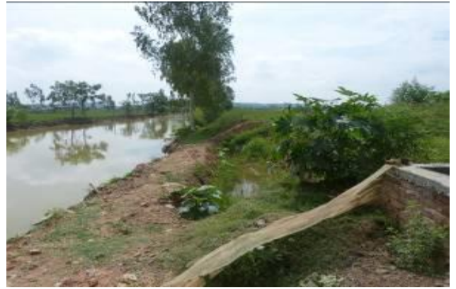
Left side of the substation adjoining the irrigation canal
