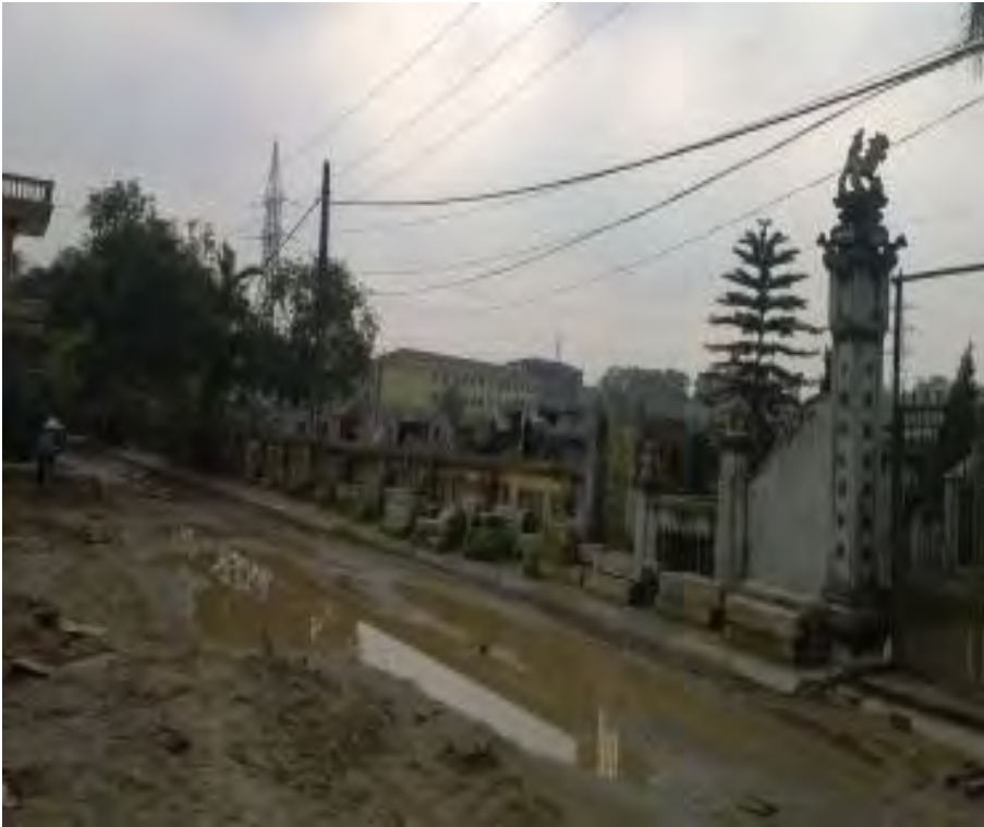
Fig 11c: OHL crossing road in Dong Ngac ward. OHL crosses local roads such as Thuy Phuong road or other inter-village/inter-commune roads.
