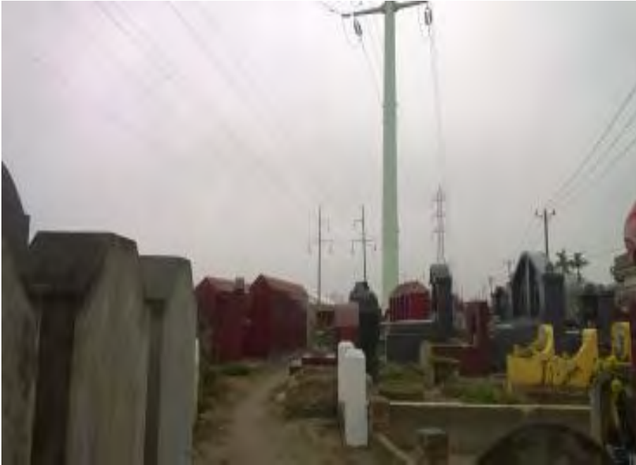
Fig 11g: The final pole for OHL is located near cemetery in Phu Thuong ward (Lane 15, An Duong Vuong street)
