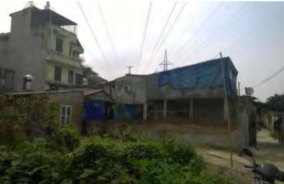
Fig 11d: OHL crosses houses in Dong Ngac ward. These houses are temporarily built and will be relocated due to the master plan of new road. The length of OHL crossing residential area in Dong Ngac Ward is estimated about 170m.
