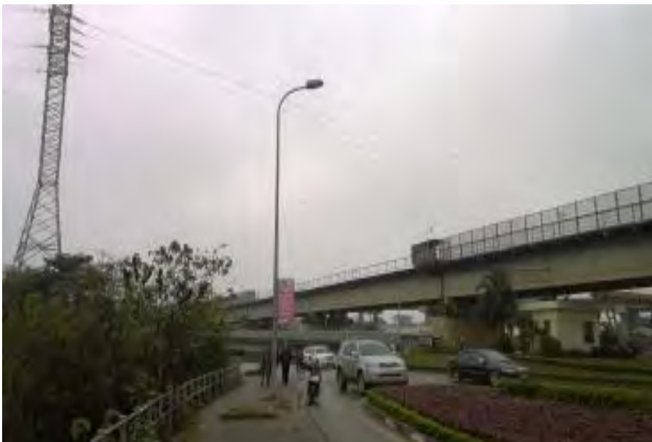
Fig 11f: The OHL crosses the Thang Long bridge, where poles are tallest (66m) to ensure transportation on the bridge
