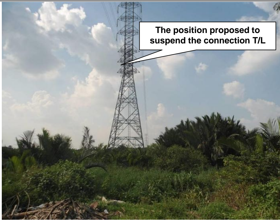
Figure 4: The existing 220kV Cat Lai - Thu Duc T/L and the position suspended the connection T/L
