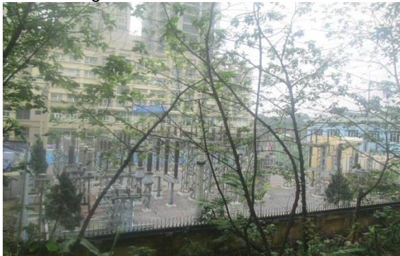
Area planned for expanding 110 kV Thanh Xuan SS
