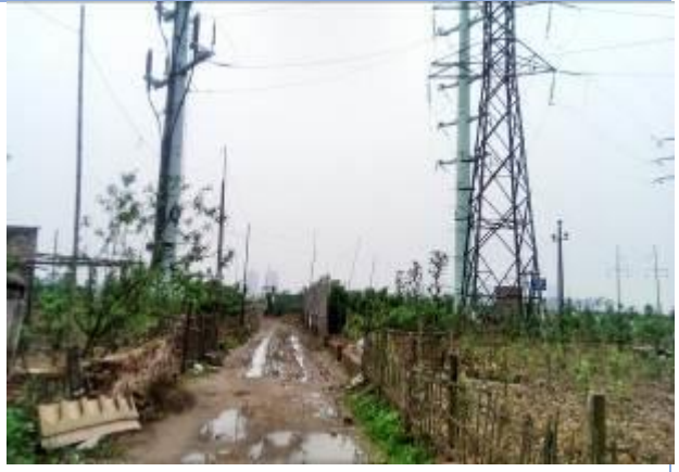
Figure 6: Expected location of underground cable
