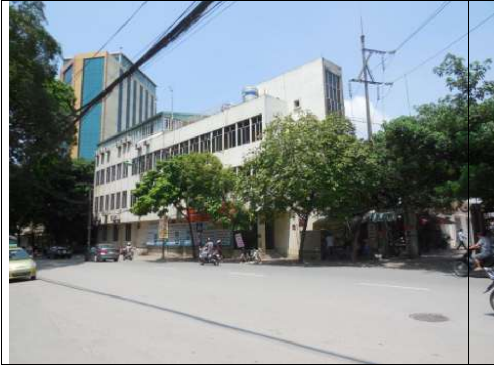
Fig 2c: Looking north at Substation from Tran Hung Dao Street
