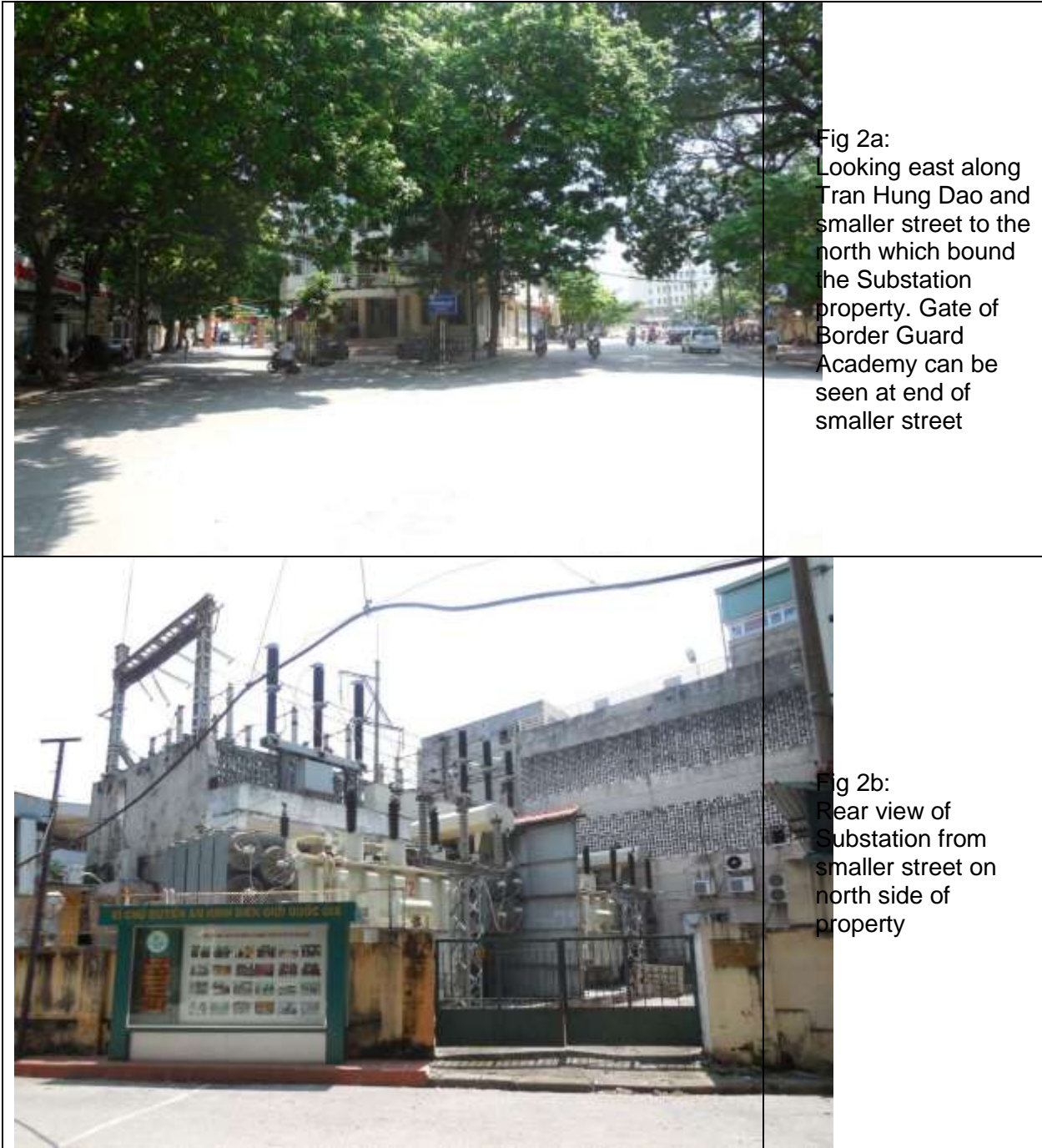
Figure 2. Views of Tran Tung Dao 110 kV Substation
