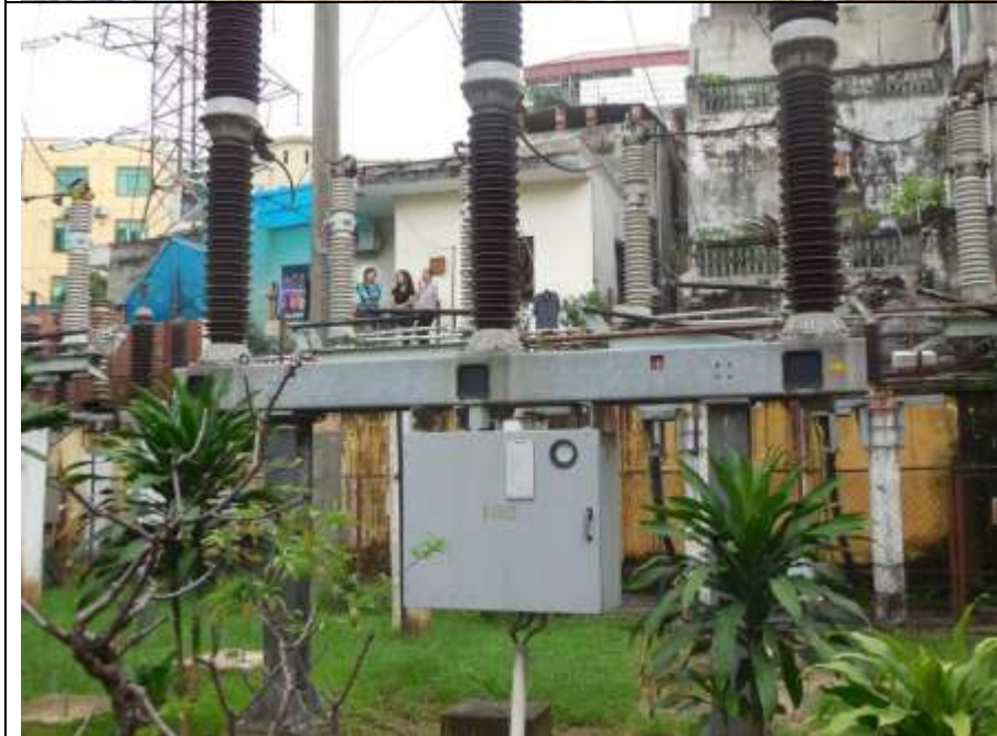
Fig 4b: View west from inside substation property showing multi- storey residences at property boundary
