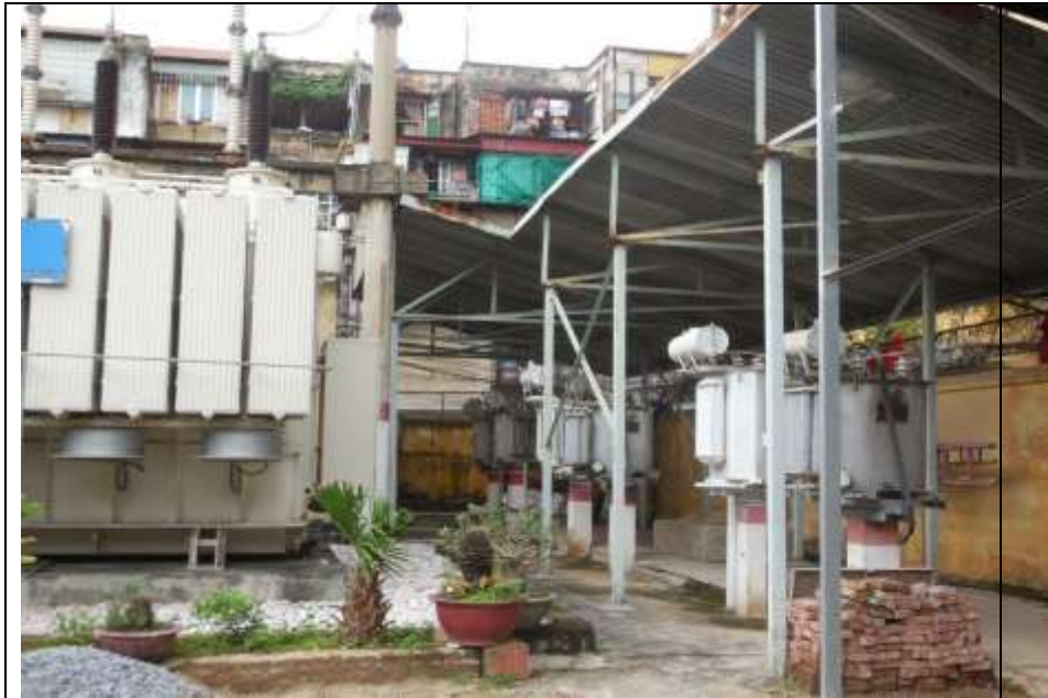
Fig 4a: View east from inside substation property showing multi- storey residences at property boundary
