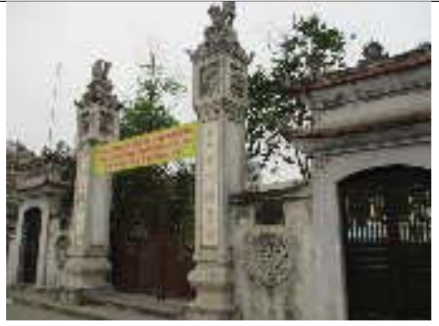
Pagoda at Frontage 5m road
