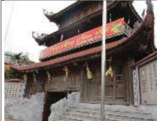
Pagoda at Frontage 5m road
