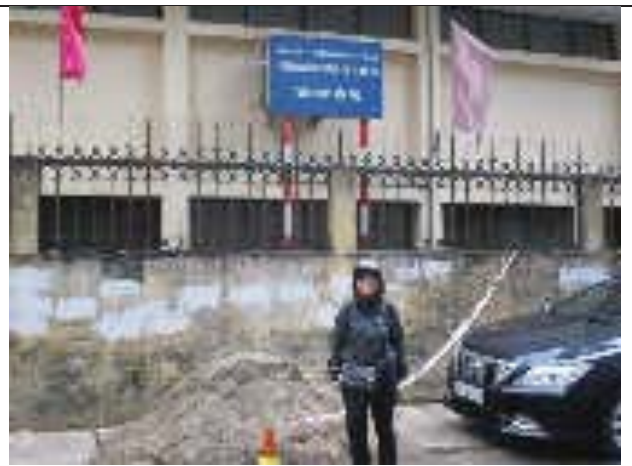
End point at 110 KW Yen Phu substation
