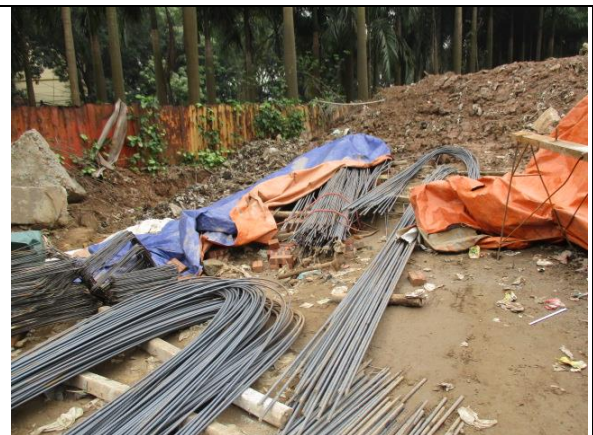
Figure 10. Building materials are not gathered neatly
