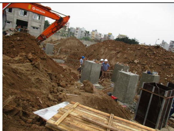
Figure 4. Excavated soil should be piled up further from construction areas
