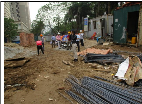
Figure 9. Building materials are not gathered neatly
