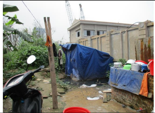
Figure 8. Toilet near the kitchen area. Around the toilet with black water backlog
