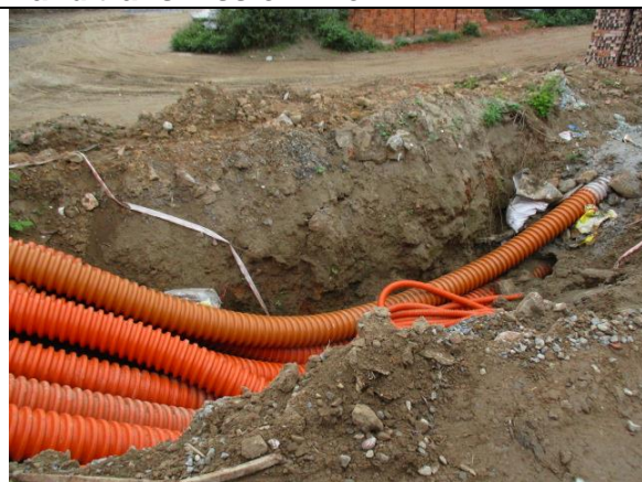
Figure 2. No warning tape/fence around
