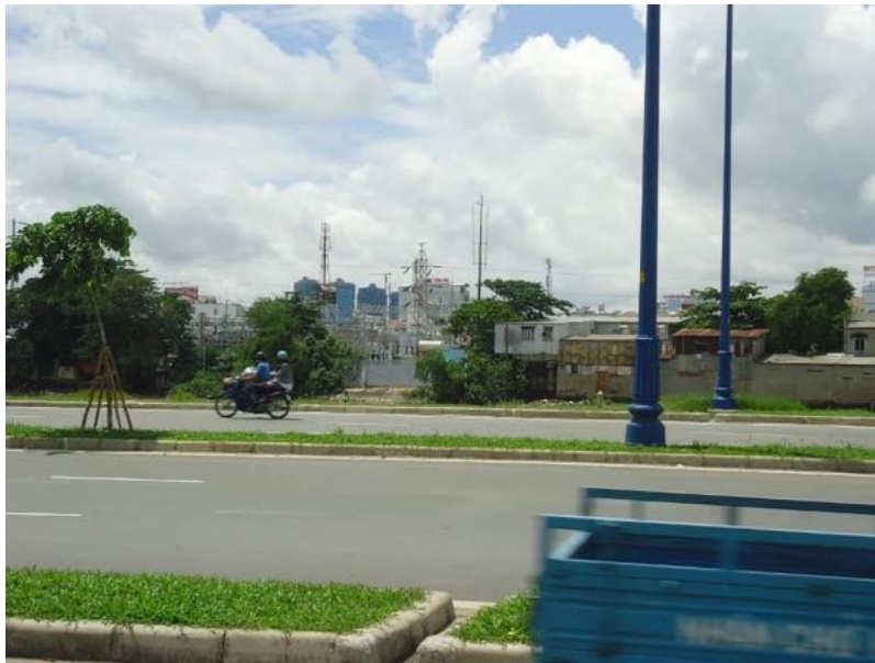
Figure 3b: The UGC section crossing under Tau Hu canal and Vo Van Kiet avenue (vision from 8-8bis Ham Tu complex).
