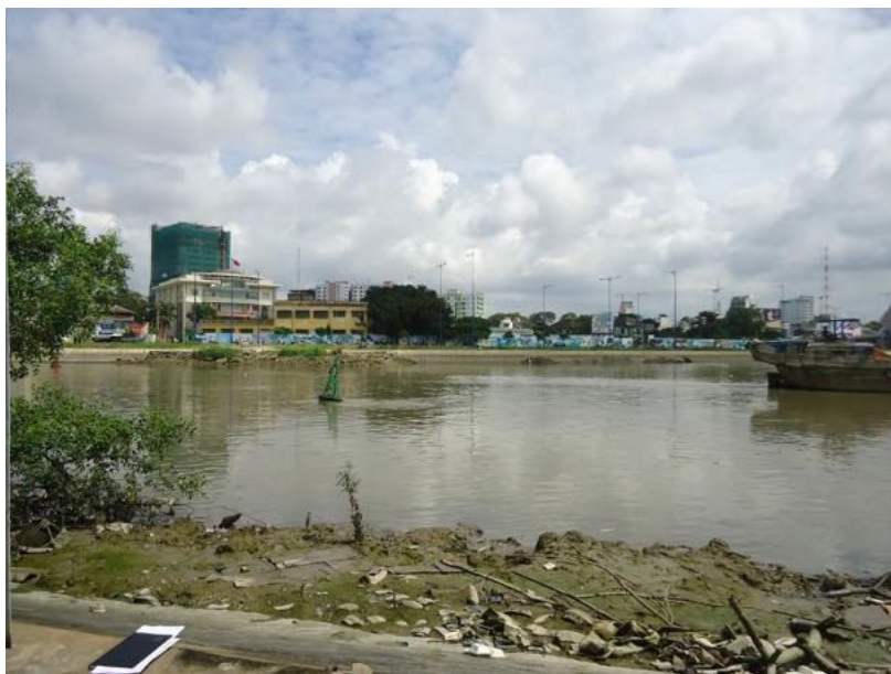
Figure 3c: UGC section crossing under canal (vision from 110kV Chanh Hung substation).
