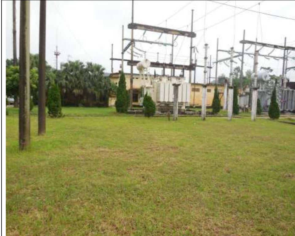
Fig 5b: Open area west of power house
