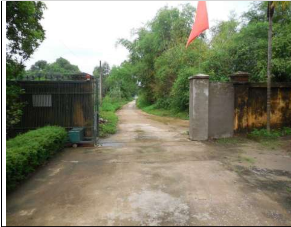
Figure 5. Views of Son Tay 100 kV Substation Property
