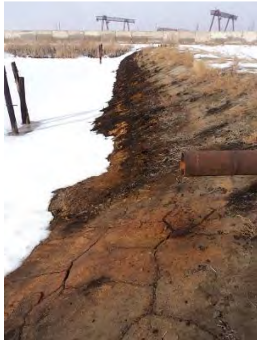
Acid waste water evaporation pond cracked and corroded concrete
