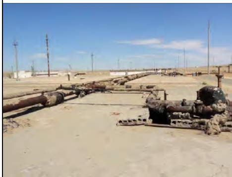
Top view of one of the groups. As it can be seen the construction material of the roof (as well as the rest of the cube) is concrete. Steam and mazut distribution pipes are disposed along the ceiling of the groups.
