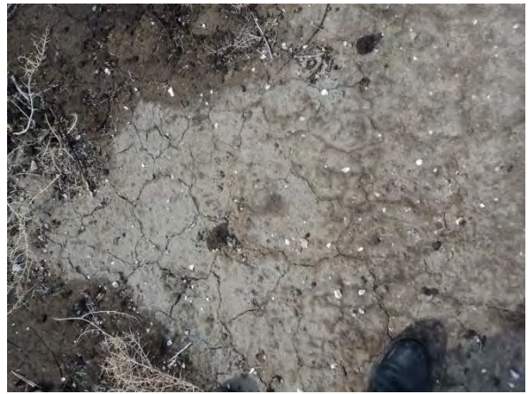
Detail of the cracked concrete material of the evaporation ponds
