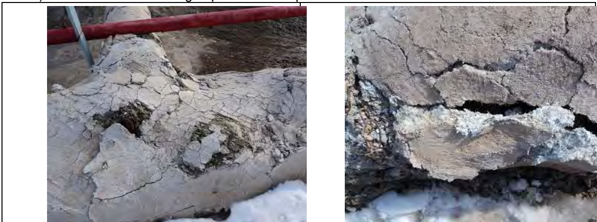
Bad condition of the pipe asbestos isolation that is exposed.
