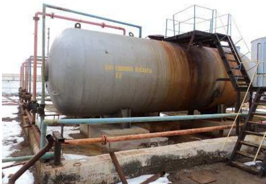
Photograph nº 18: Impervious secondary containment for chemical tanks
