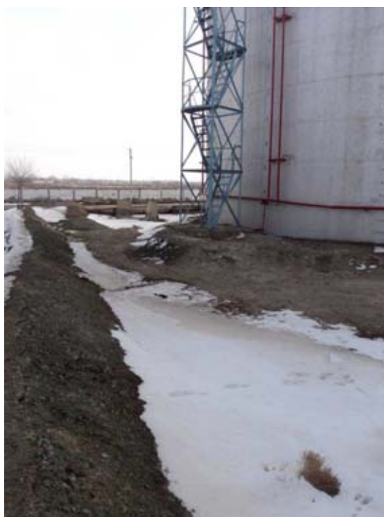
Photograph n° 11: Mazut secondary containment material is soil. No impervious material.
