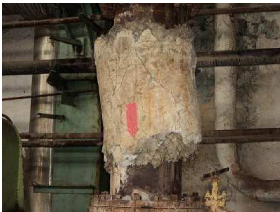
Photograph nº 48: Bad condition of the pipe asbestos isolation that is exposed to the open.
