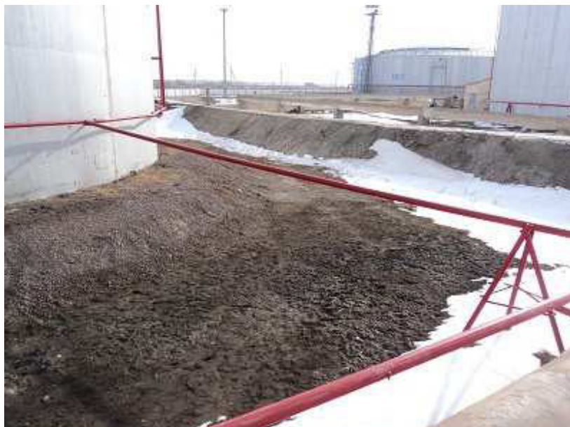
Photograph n°12: Mazut spot over the soil basement.
