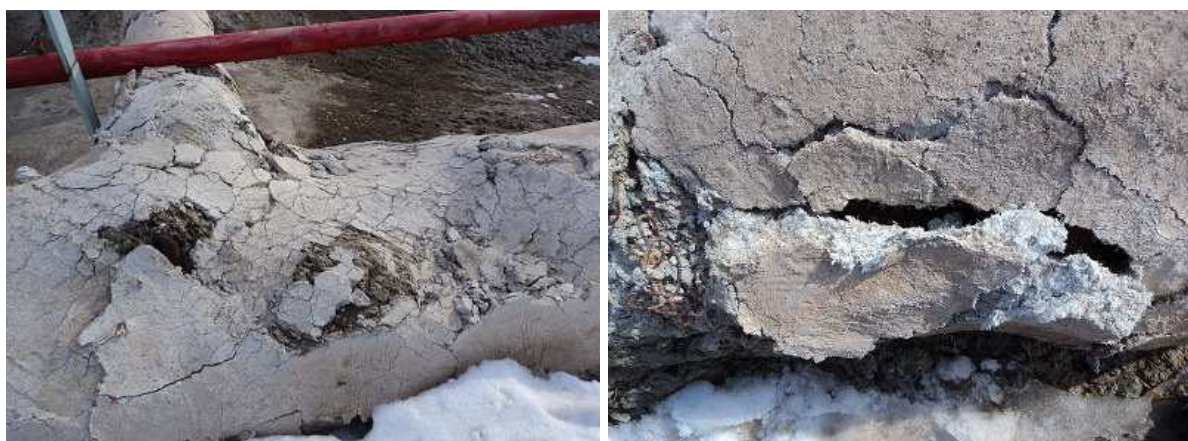
Figure 26. Bad condition of the pipe asbestos isolation that is exposed.
