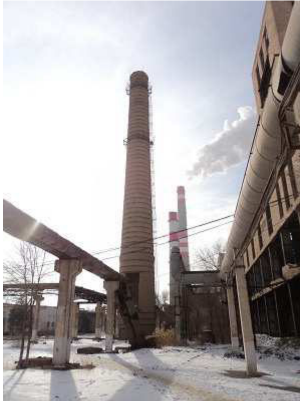
Photograph n° 8: First stack is the remaining stack of the dismantled units I and II. Second stack is the stack of units III and IV to be decommissioned. Third stack is the stack of units V and VI that will remain.
