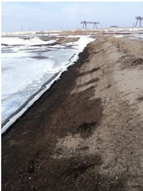
Figure 21. Oily waste water evaporation pond
