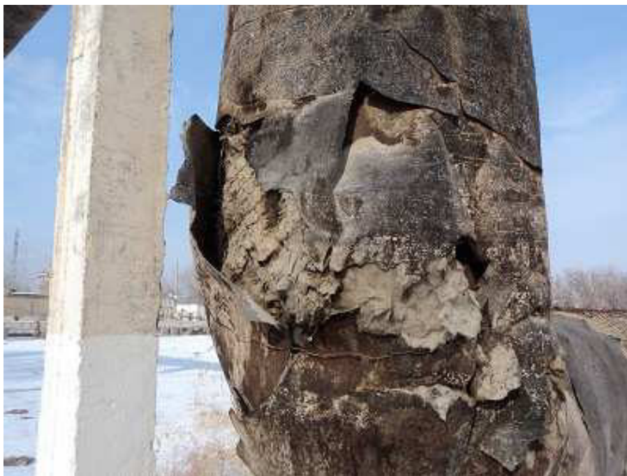
Photograph n° 45: Bad condition of the pipe asbestos isolation that is exposed to the open.
