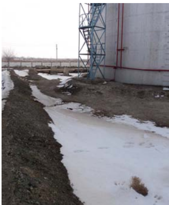
Figure 27. Mazut secondary containment material is soil. No impervious material.
