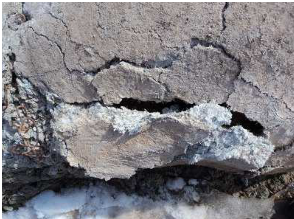
Photograph nº 47: Bad condition of the pipe asbestos isolation that is exposed to the open.
