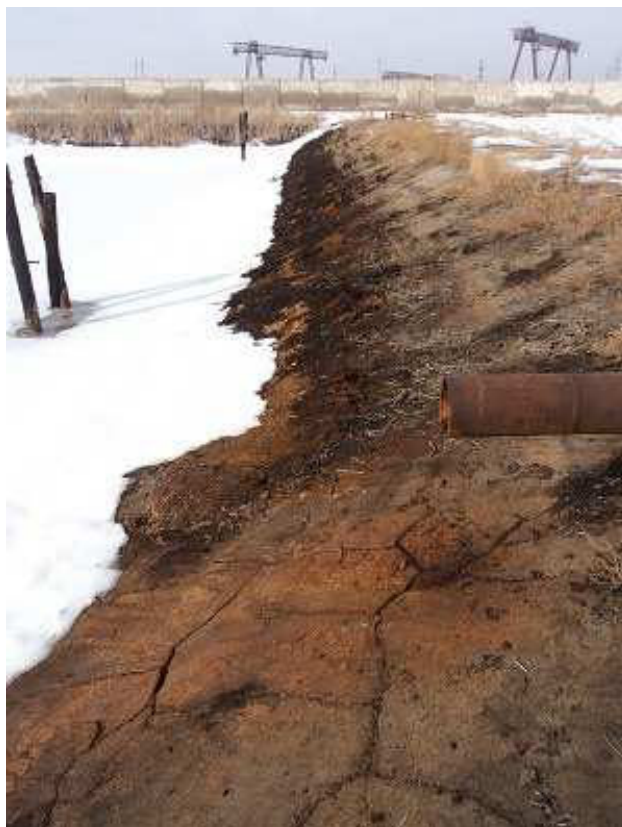
Photograph nº 32: Acid waste water evaporation pond cracked and corroded concrete
