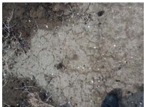
Figure 22. Detail of the cracked concrete material of the evaporation ponds
