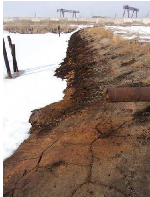
Figure 24. Acid waste water evaporation pond cracked and corroded concrete
