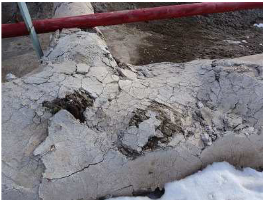
Photograph n° 46: Bad condition of the pipe asbestos isolation that is exposed.
