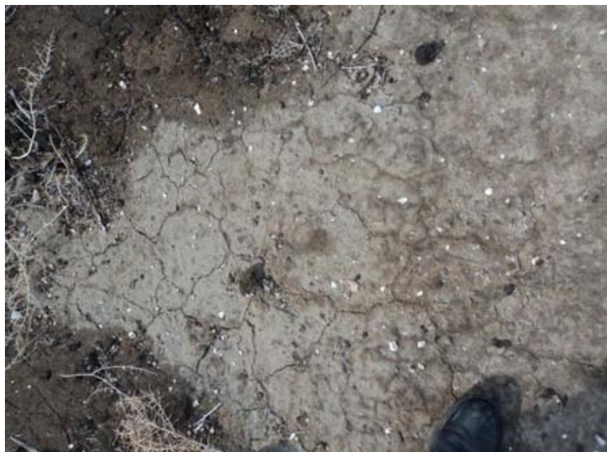
Photograph nº 30: Detail of the cracked concrete material of the evaporation ponds.
