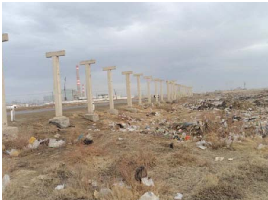
Photograph n° 43: Municipal landfill used by the TPP for its solid waste disposal. Landfill doesn't include an impervious layer or other prevention pollution measures. Close distance to the TPP can be observed
