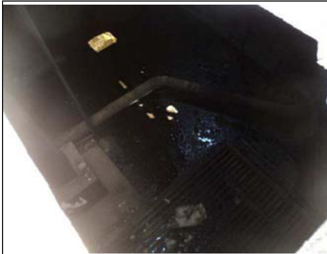
Interior view of one of the tanks from the top. A layer of residual mazut can be observed.
