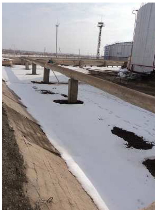
Photograph n° 13: Mazut secondary containment concrete walls are in bad condition. Basement still made of soil.
