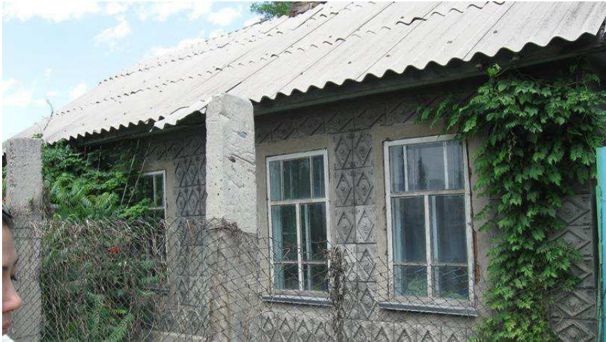
Project Affected House
