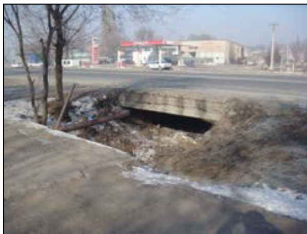
Flood canal in Novo-Pavlovka Village
