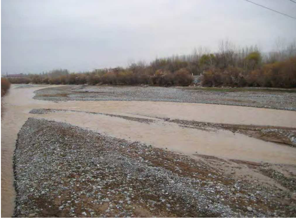
Fig. 3: River Kugart at the location where it is crossed by the Project road
