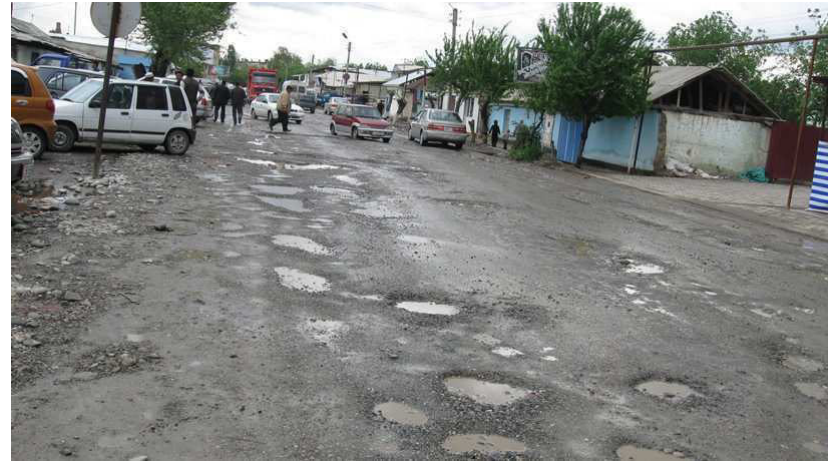
The existing road condition
