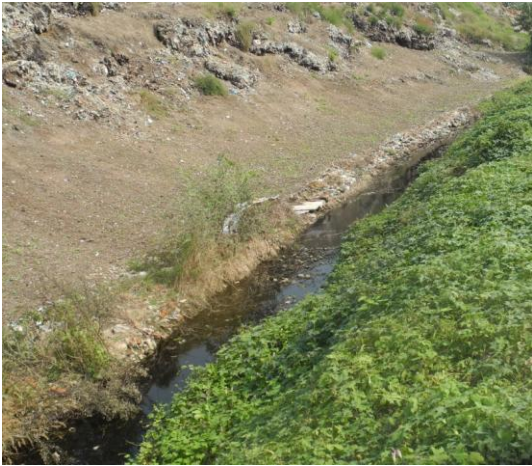
Drainage Channel around the Landfill (1)
