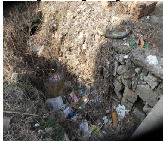
Existing Sundian Drainage Channel
