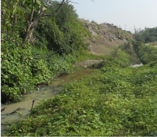
Drainage Channel around the Landfill (2)
