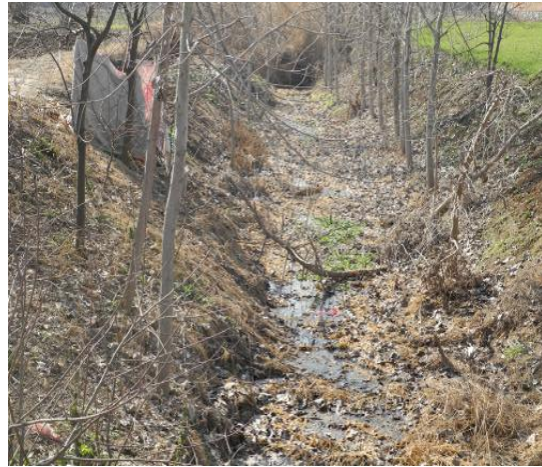
Existing Chenxiang Drainage Channel
