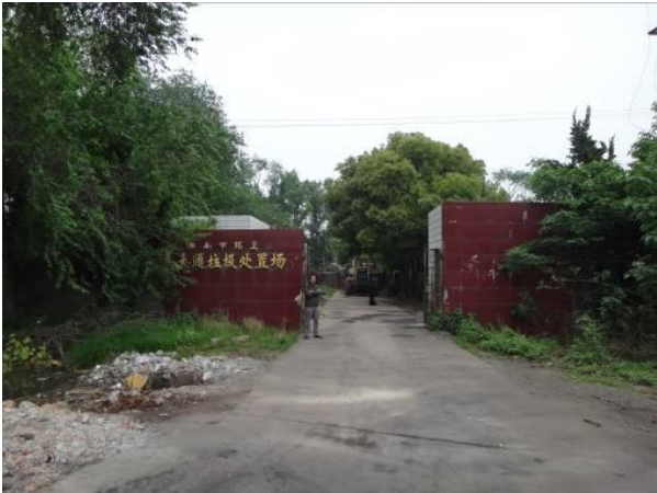
Management Area of Datong Landfill
