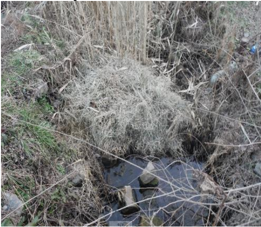
Existing Datong Drainage Channel
